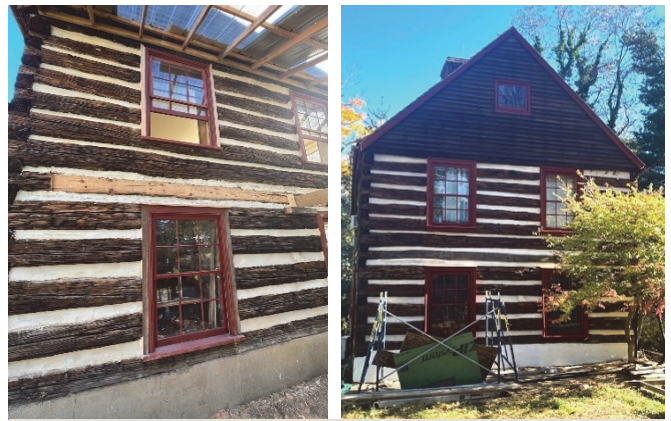
Close-up of the newly installed 19th century windows (left); completed restoration of the gable end facing the parking lot (right).
