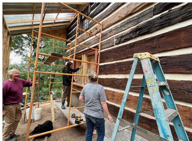
Stroik trained and enlisted Stenton staff in helping with daubing and other tasks. Note the replaced logs (lighter in color).
