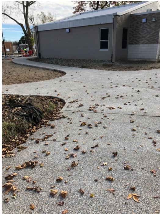
Figure 4 - Current conditions of Grid 1, facing southwest
